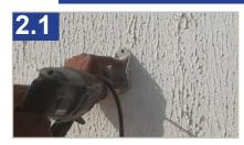
Place the Stand Base U-shaped Clamp vertically, then mark the holes to drill;
