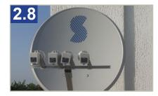
Insert 1\*LNBF in each mounted LNBF Clamp;
