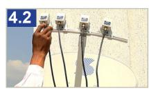
Use the 4\*RG-6 coaxial cable runs to connect the LNBFs to the switch:
