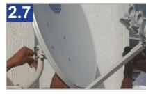
Mount the Reflector assembly onto the Stand Pole and tighten the 4\*M6 Nuts on the Pole Clamps;
