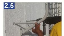
Align the Side Legs to obtain a perfectly vertical Stand Pole (using an inclinometer or level gauge), mark the holes to drill;
